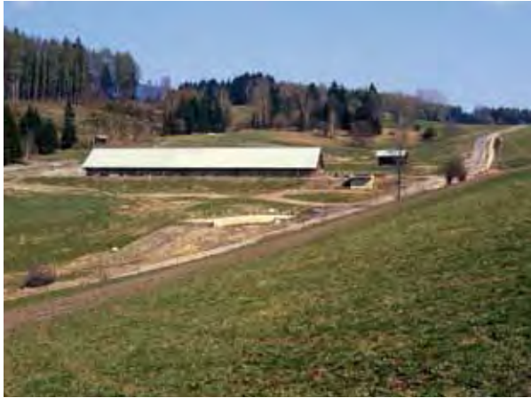
At the end of the last century a large calf-raising facility was built in close proximity to the valuable botanical locality at Bíner. This irresponsible act was at the expense of many hectares of species-diverse wetland meadows, which were unprotected at the time, but are now, thankfully, under the strict protection of the European Union (photo Jan Štursa)
