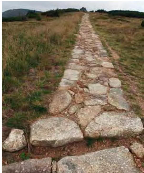
The trail to Mt. Harrachovy kameny is relatively narrow and paved with granite blocks. It replaced a wider, gravel trail (2011, photo Kamila Antošová)
