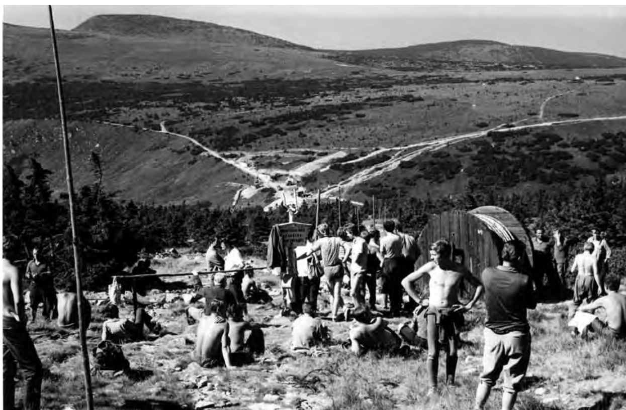
Laying cables from the Labská bouda Chalet to Martinova bouda and to the Sněžné jamy Cirques, probably in 1969. As with Mt. Sněžka the electric cable and water mains run from the Polish side, while the cable to the Sněžné jamy Cirques runs from the Czech side. Connecting Krkonoše to mains electricity and water has continued from 1965 until today. During these works the surface cabling has been replaced and nearly all of the previously unconnected localities have been electrified (of the large enclaves, the Klínové Boudy Chalets was connected in 2008). We must also mention the lines of telecommunication cables. Linear constructions are a sensitive matter, which are still carefully monitored (photo Miroslav Hladík)
