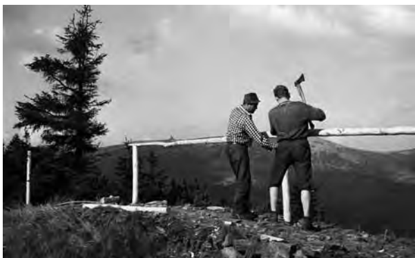
In addition to repairing the trails, effective measures were also taken to direct the movement of tourists. Here the Administration staff are building the Šmíd Vantage Point on the eastern slopes of Krkonoše. 1960s (photo Miroslav Hladík)
