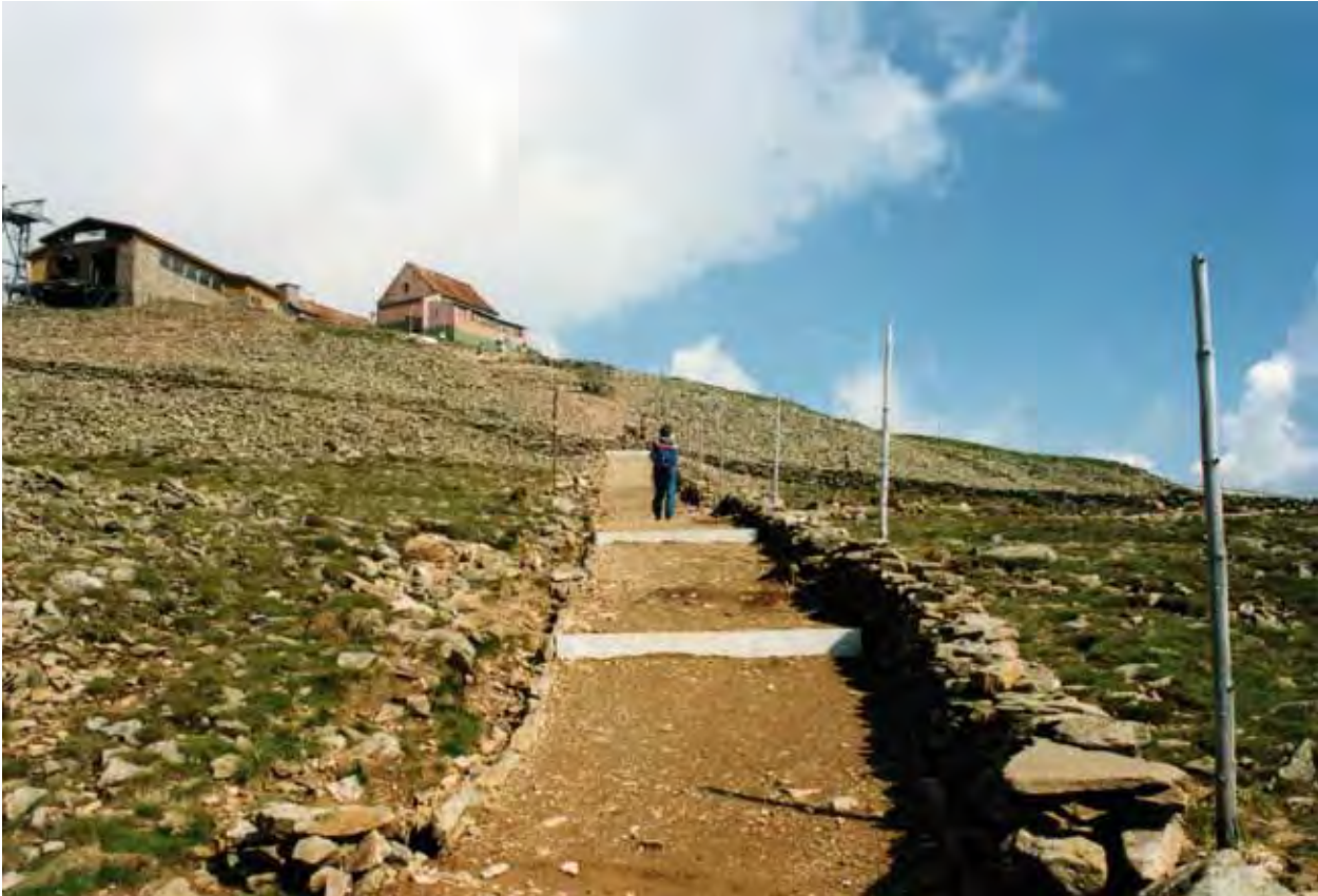
The overall appearance of the repaired trails is improved by the lateral stone walls, which are also effective in the fight to keep the tourists from straying away from the trail (this is the First Zone of the national park, with the strictest protection regime). The Česká bouda Chalet is still standing... (photo Jan Štursa)
