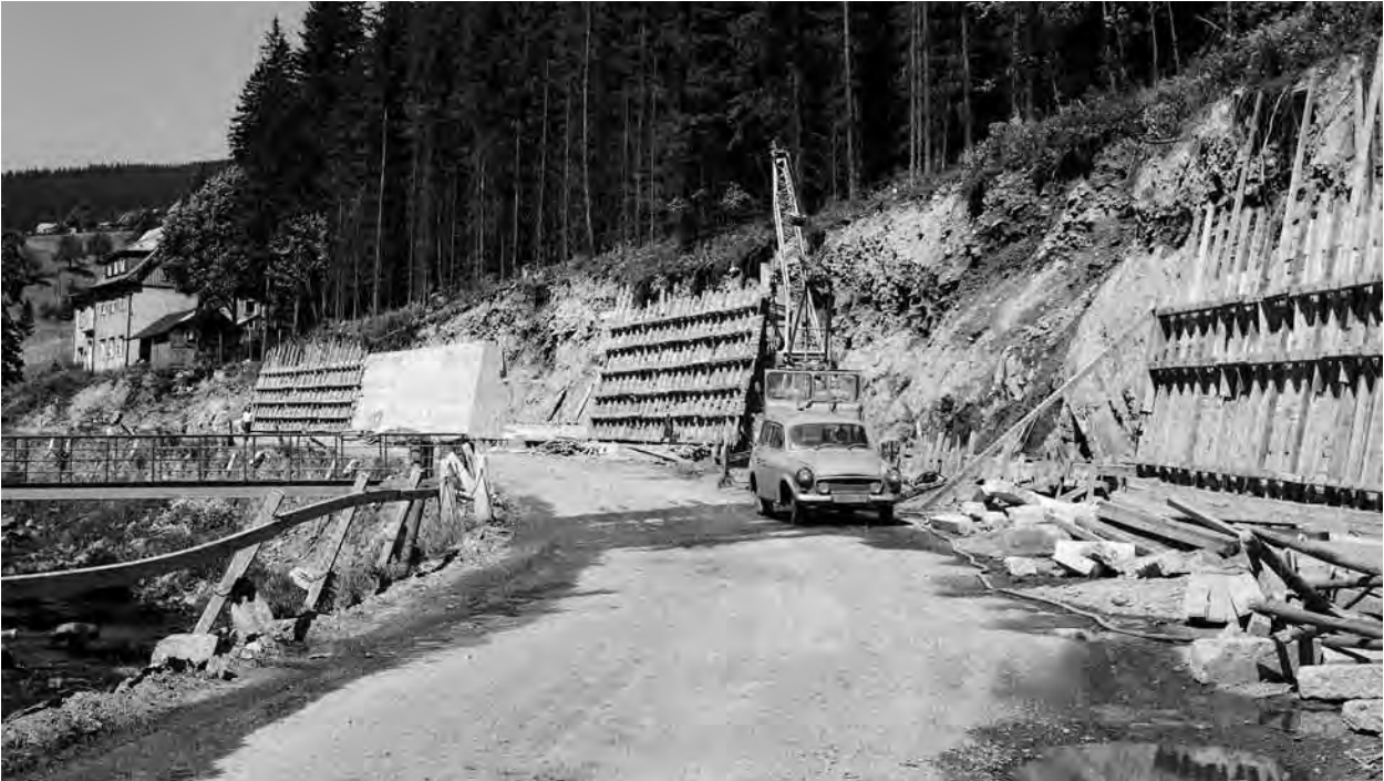
The series of reconstructions of main roads leading to the Krkonoše resorts and to the border crossings was begun in 1969. By 1979 the Horní Maršov—Pec pod Sněžkou (depicted here), Vrchlabí—Špindlerův Mlýn, Temný Důl—Pomezní Boudy and Kořenov—Harrachov roads were gradually widened by Polish construction companies. Later the Harrachov bypass was built – the more unnecessary the road, the wider it was built! (photo Miroslav Hladík)
