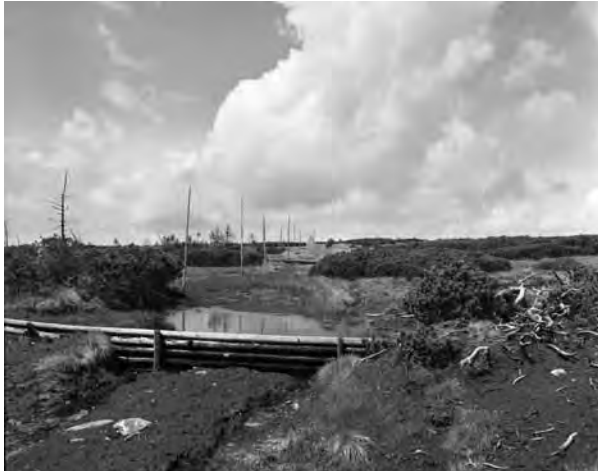
Barriers on the former trail between the Labská and Vosecká bouda Chalets prevent erosion caused by trampling the waterlogged terrain and contribute to the stability of the water regime on the Pančavské rašeliniště Peatbog (1995, photo Karel Hník)
