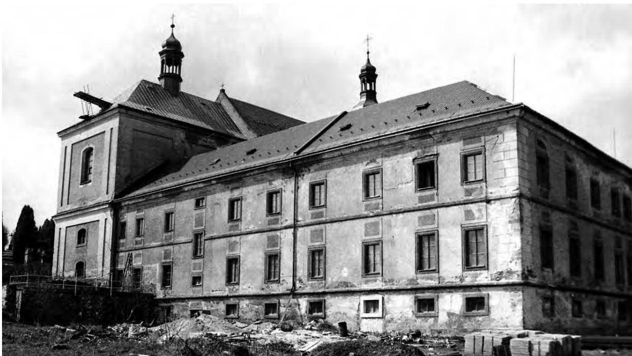
Since the 1950s the Museum of Krkonoše in Vrchlaví has occupied the Augustinian Monastery building. The KRNAP Administration took control of the museum in 1966 and carried out a demanding renovation project, which dragged on for 17 years (photo Jiří Bruník)
