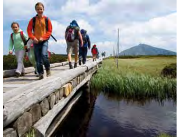
In place of the former limestone embankment, an oak-built wooden walkway runs across the revitalized Úpské rašeliniště Peatbog on piles (2009, 13 years after it was built, photo Kamila Antošová).
