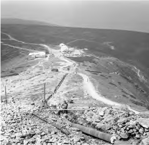
Combined trench for water pipes, electricity and telephone cables, 1974. Although the shallow trench was covered with rocks, it can be seen clearly again today (photo Jan Štursa)
